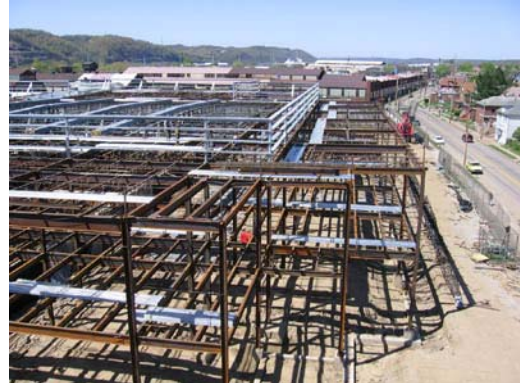
Structural Steel Erection Complete Composite Deck Placement Beginning
