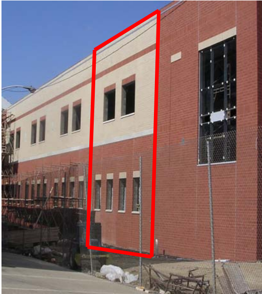
Conventional brick and CMU façade as built with area of precast panel outlined.
