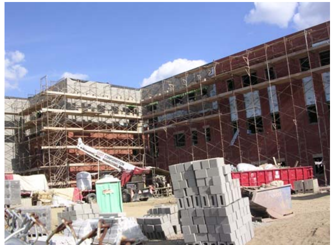
Mason scaffolding around building footprint.
